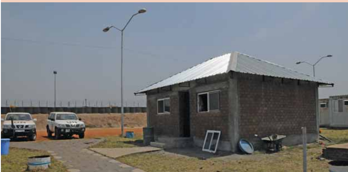
Soil blocks have been used to build houses such as this one at an UNMISS base in Juba, South Sudan, based on good practice from Darfur
