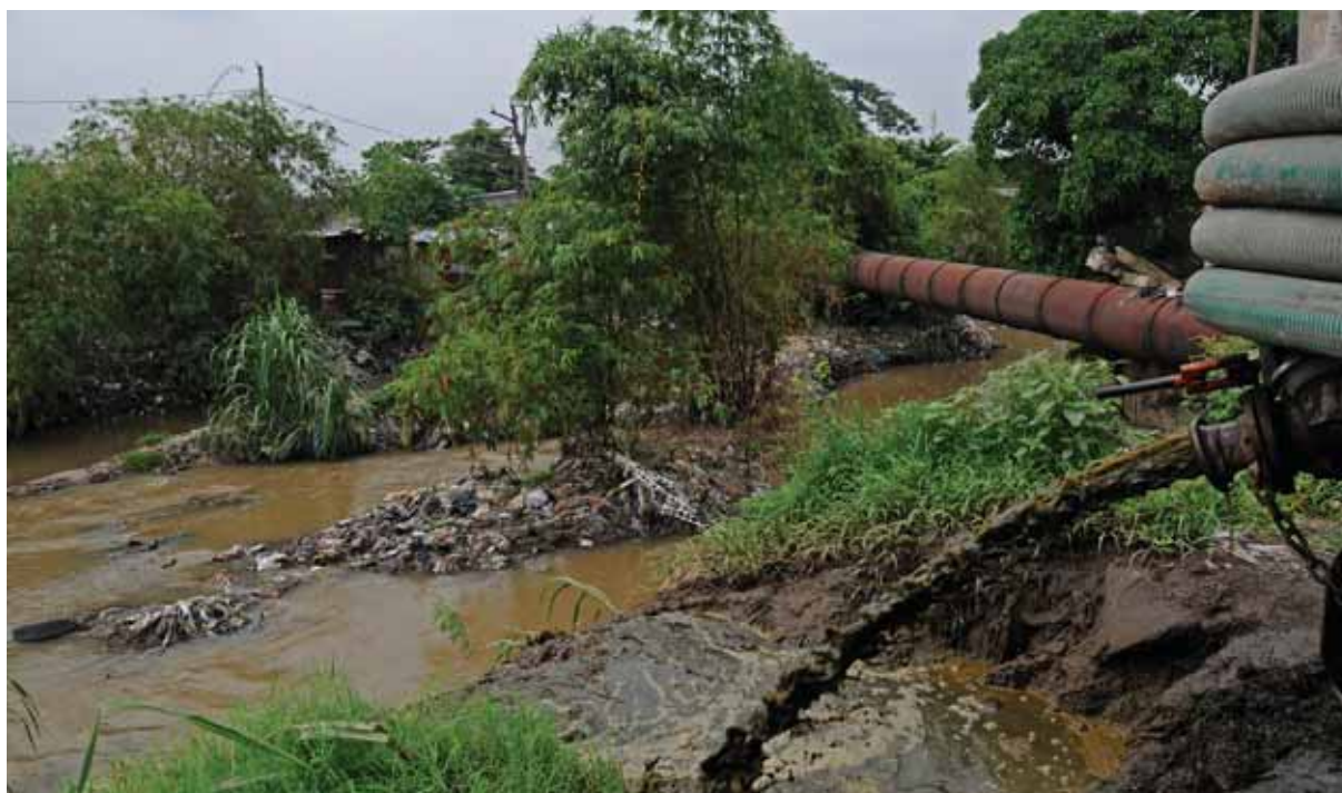
Unsanitary sewage disposal site near Kinshasa in the DRC, 2009
